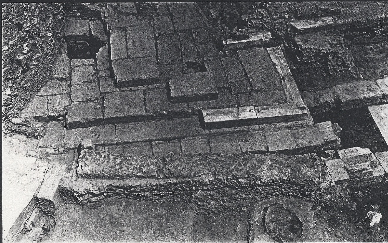
Fig. 3 Marble-stepped platform of poros blocks built against southwest corner of temple
